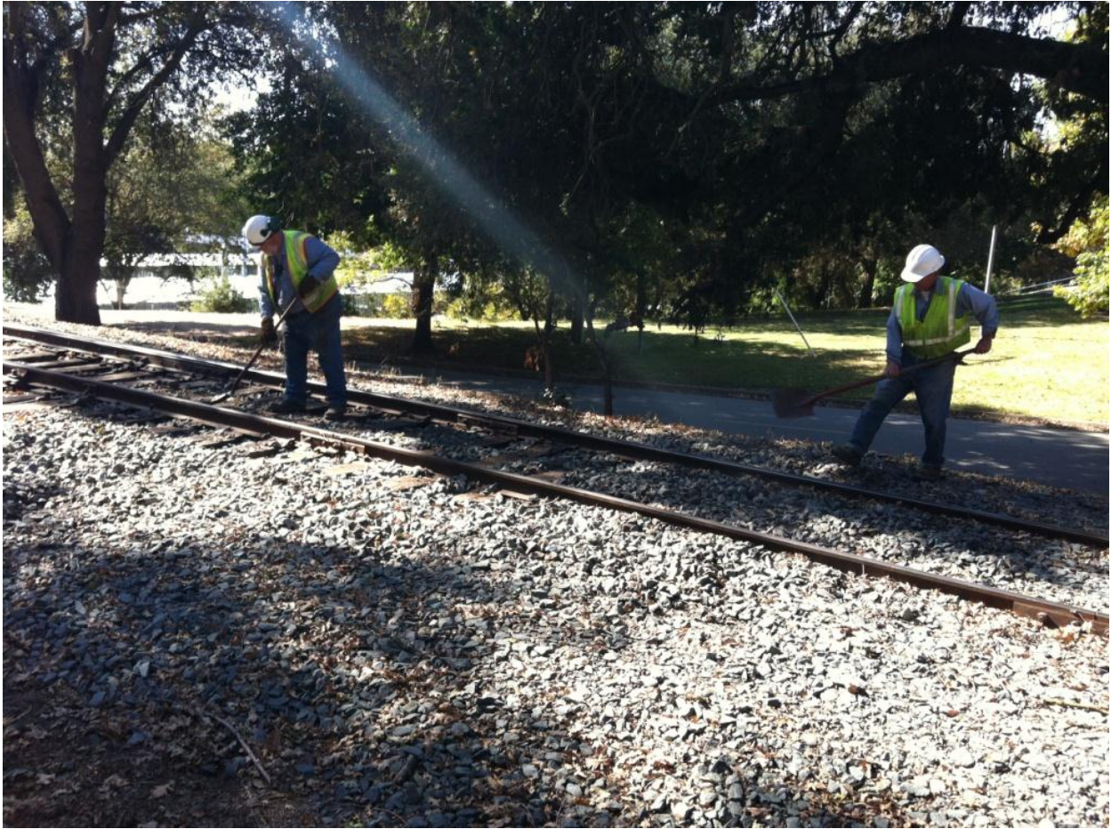
At Switch 14, North Miller, Frank and Mike T. shovel rock into the “dip”
