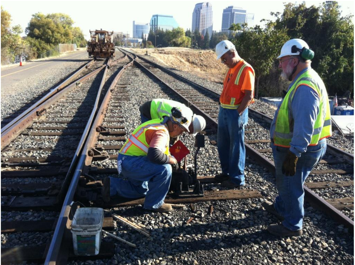
Mike F., Clem, John, and Frank make adjustments to the ground throw switch at Clunie
