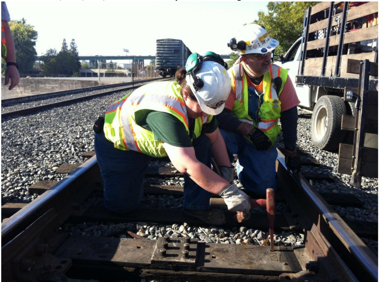
Heather and Mike F. work on resetting the gauge plate of Switch 13 at Clunie
