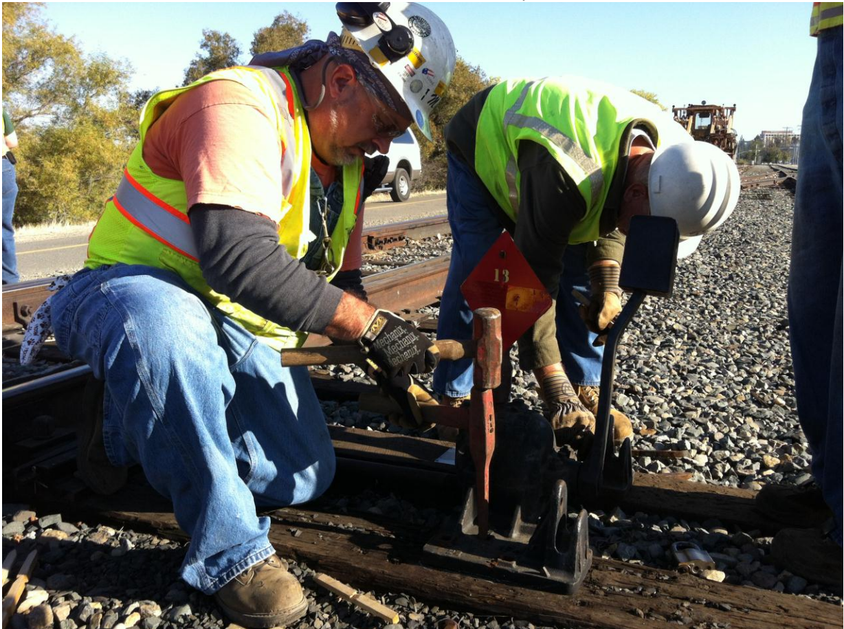
Mike F. and Clem set and re-spike the ground-throw switch at Clunie
