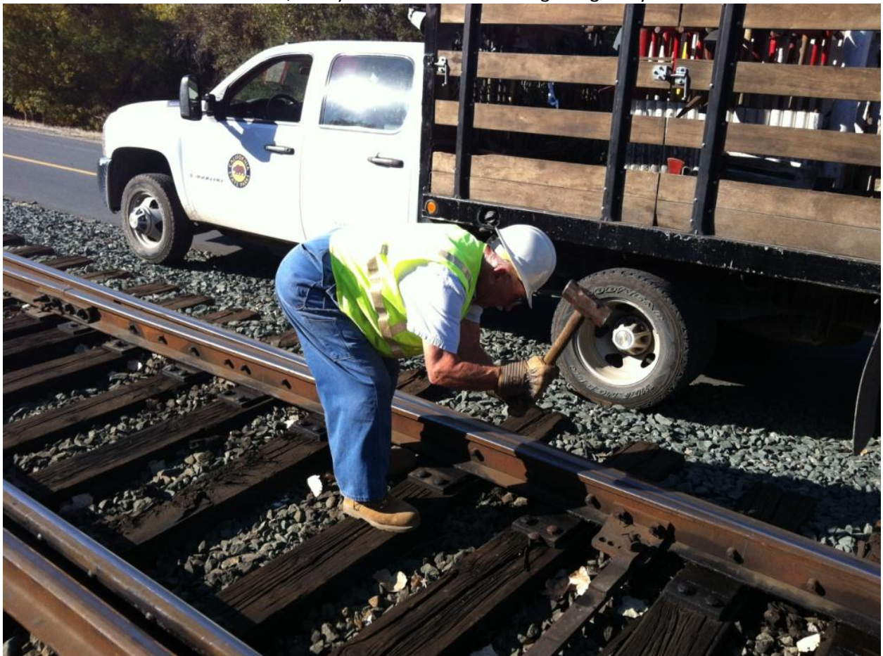
Clem re-spikes switch plates
