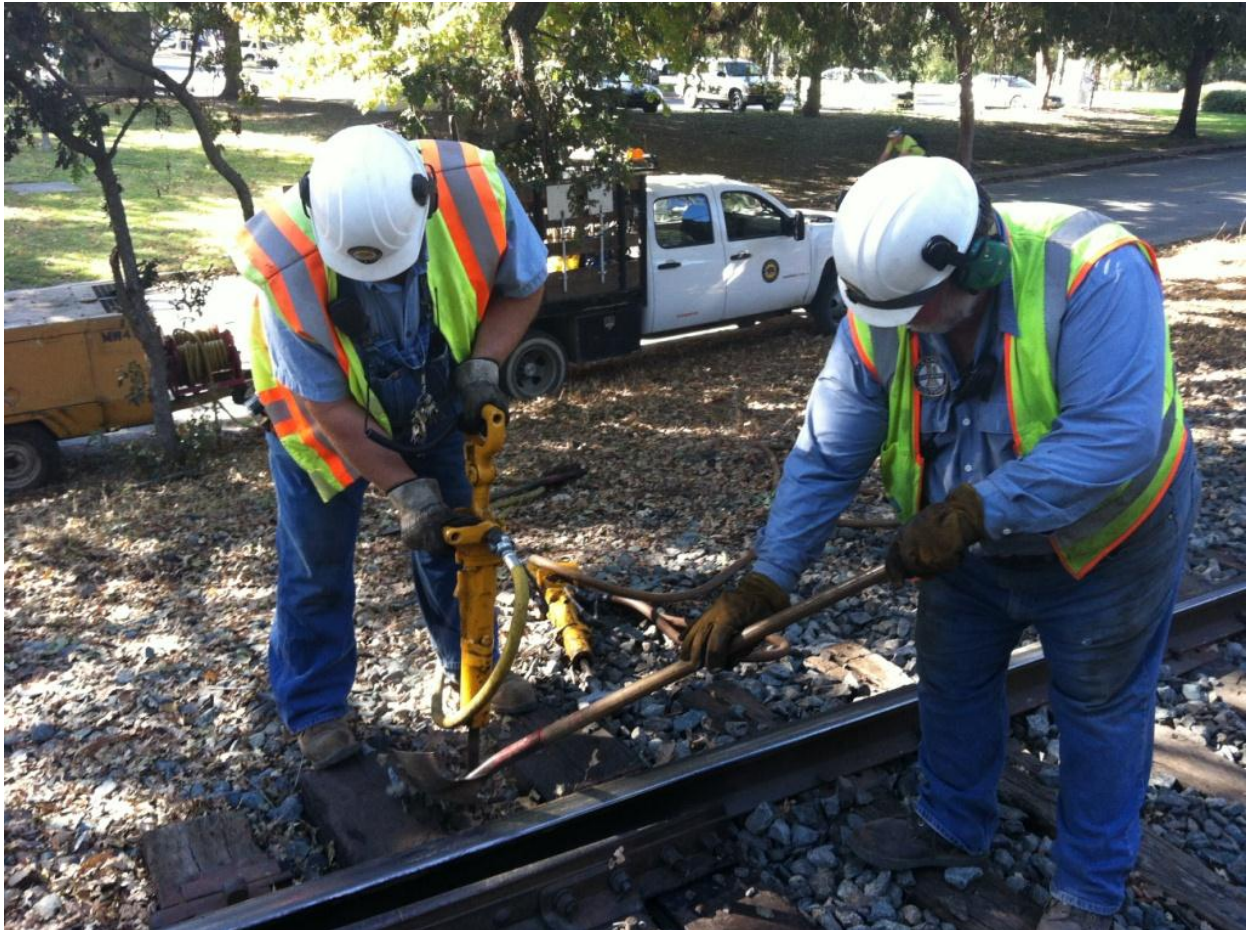
Chris uses the pneumatic hand-tamper while Frank shovels in rock
